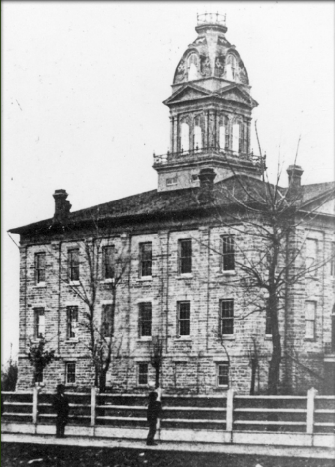
Kankakee County's Second Courthouse, built 1873.
